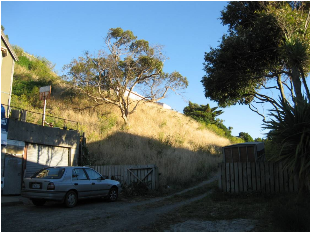
View from Princess Terrace to rear of Housing Property (vehicle parked outside 27 Princess Terrace)
