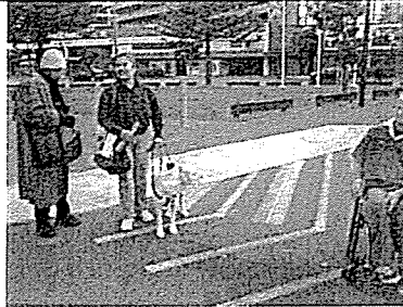
No provision of tactile indicators to assist with direction for crossing
