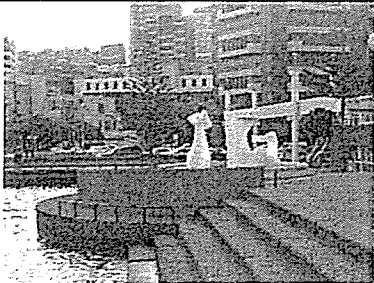
Non continuous barrier where there is a fall of 1m or greater into the water
