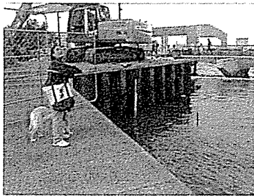
2m+ Drop into shallow water with no barrier or indication that it is present.
