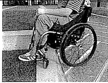
Large saw cuts that catch chair wheels and dismount users trying to access grass areas.
