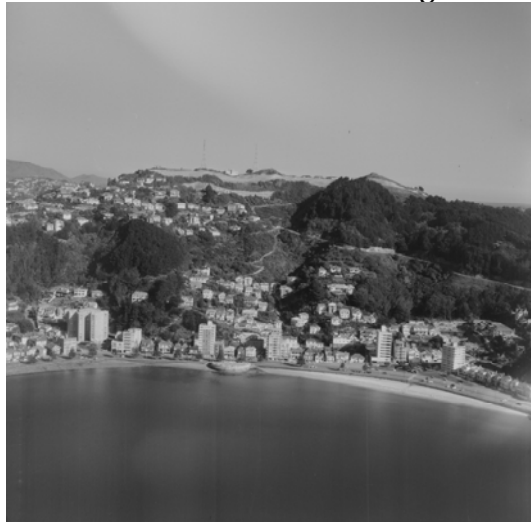
Figure 14: View of Mt Victoria over Oriental Bay, 1965. The summit area typifies the pressure of use on the Town Belt’s high points. Pictured are radio masts and the broadcasting station above the new road works cut to construct Lookout Road and complete the ridgetop scenic drive along Alexandra Road. Interestingly, there was little protest at the time about the visual impact of this roading development.
