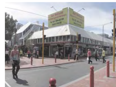
Figure 23. Existing address to Cuba Mall.
