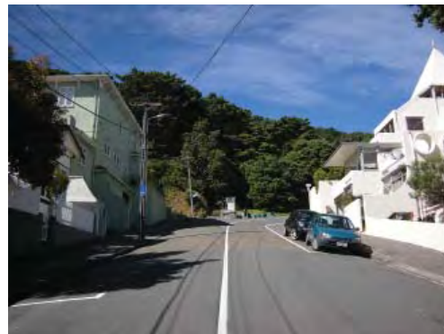
Figure 10. Existing Majoribanks Street.
