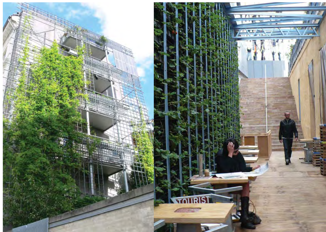
Figure 25. Retrofitted green walls and roofs can be introduced to deliver some benefits for both the performance of buildings and public amenity.
