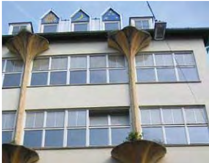
Figure 37. Innovative ways to provide green infrastructure within buildings will be investigated, the example above slows the water on its path to the stormwater system by using planting.
