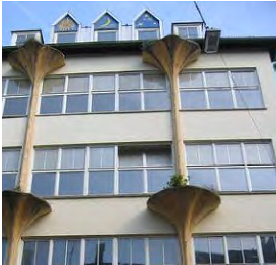
Figure 37. Innovative ways to provide green infrastructure within buildings will be investigated, the example above slows the water on its path to the stormwater system by using planting.
