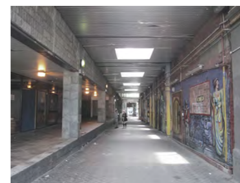
Figure 13. Existing Opera House Lane.
