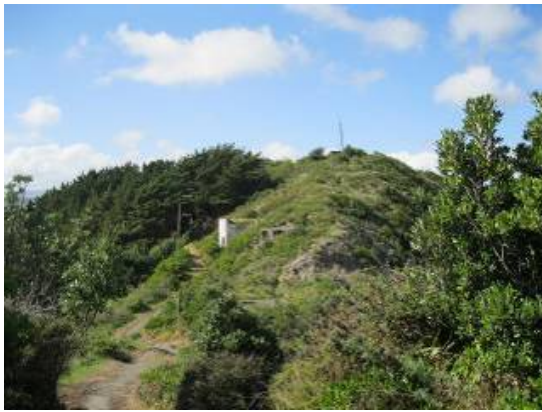
Telecommunications tower on the ridgeline
