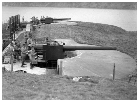
1937 photo of original 6-inch gun emplacements positioned facing south over the harbour entrance.
