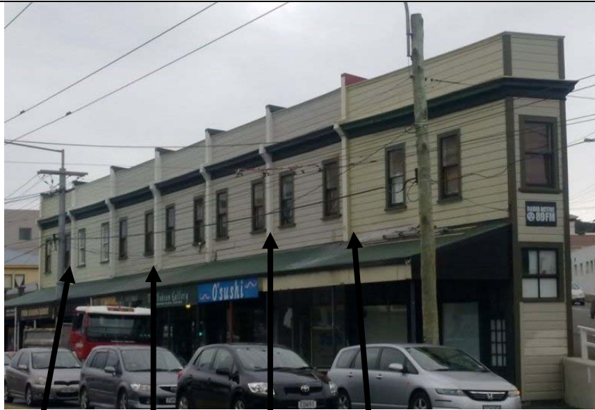
Unreinforced brick walls between each shop (and residential) unit and at one end (overleaf).
