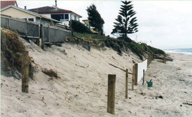
June 1997: eroding dune prior to replanting.
