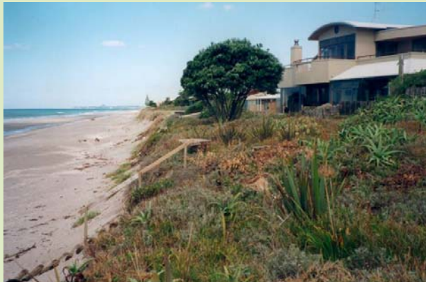
Houses too close to sea
