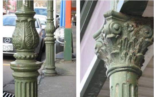
Detail of cast iron veranda posts
