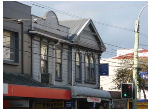
Upper level windows and parapets
