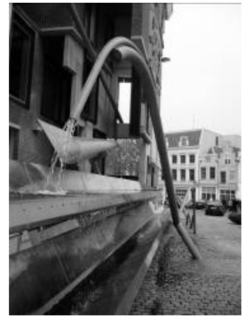
Richness of detail at ground level
