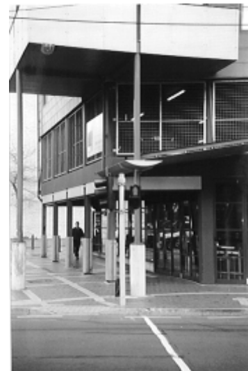
Building frontage to the street
