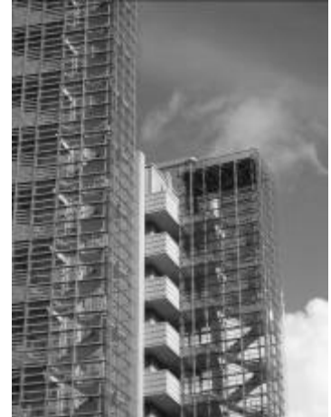
Sophisticated detailing in a contemporary building
