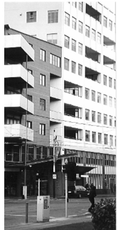
Complementing an existing building
