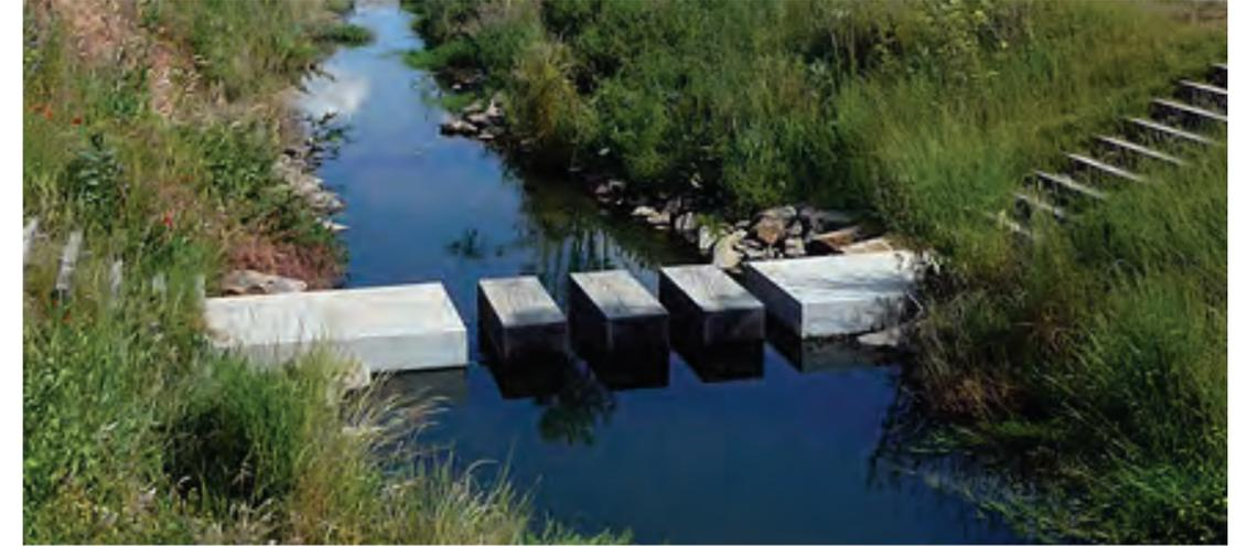
Connection to the water, function to capture debris also
