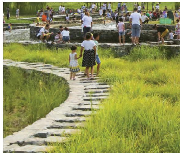
Low wall at stream edge to control flooding
