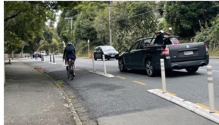
Figure 7: Existing physical separators prevent vehicles from casual encroachment
