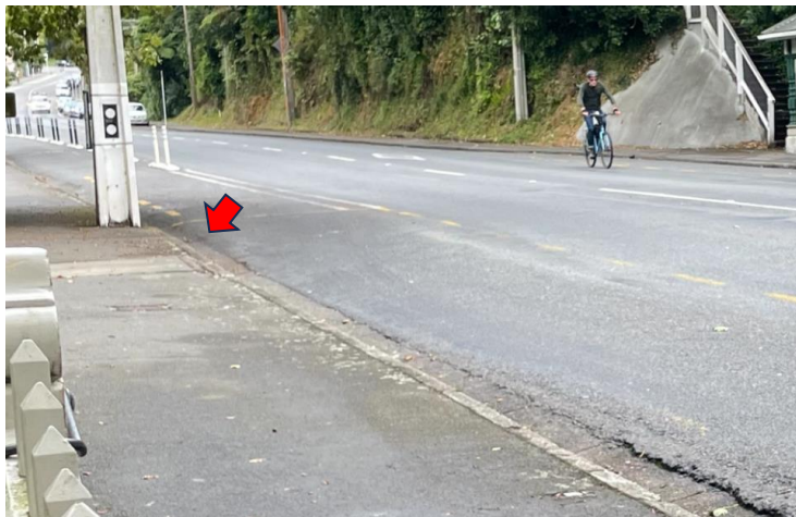
Figure 6: When measuring effective width of the cycleway, the deep stormwater channel (red arrow) is not rideable space
