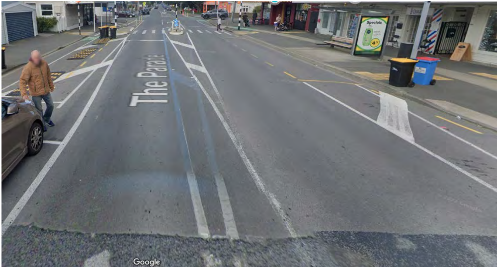
[The parade - Island bay] Visually chaotic road with old markings still showing
