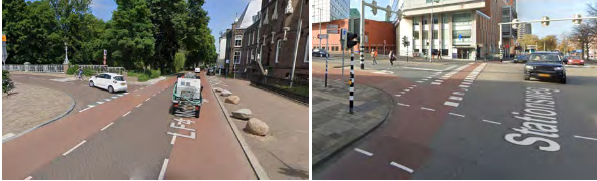
[LF4 Midden - Utrecht (left), Stationsweg - Groningen (right)] Continuous red asphalt bike lane intersections on a quiet and busy road, with clear give-way “shark’s teeth” markings.
