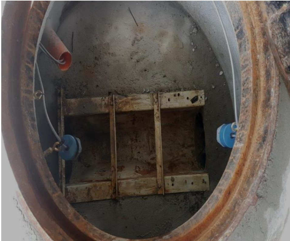
Photo 2: View down a manhole of a wastewater overflow pipe that redirects excess wastewater from a pump station into a stormwater pipe. The stormwater pipe discharges into a nearby stream (Source: WWL response to further information request email dated 4 May 2018).
