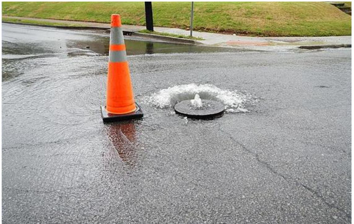
Photo 3: View of a manhole overflowing onto the street and discharging into the stormwater network via nearby curb and channel/sumps (Source: WWL response to further information request email dated 4 May 2018).
