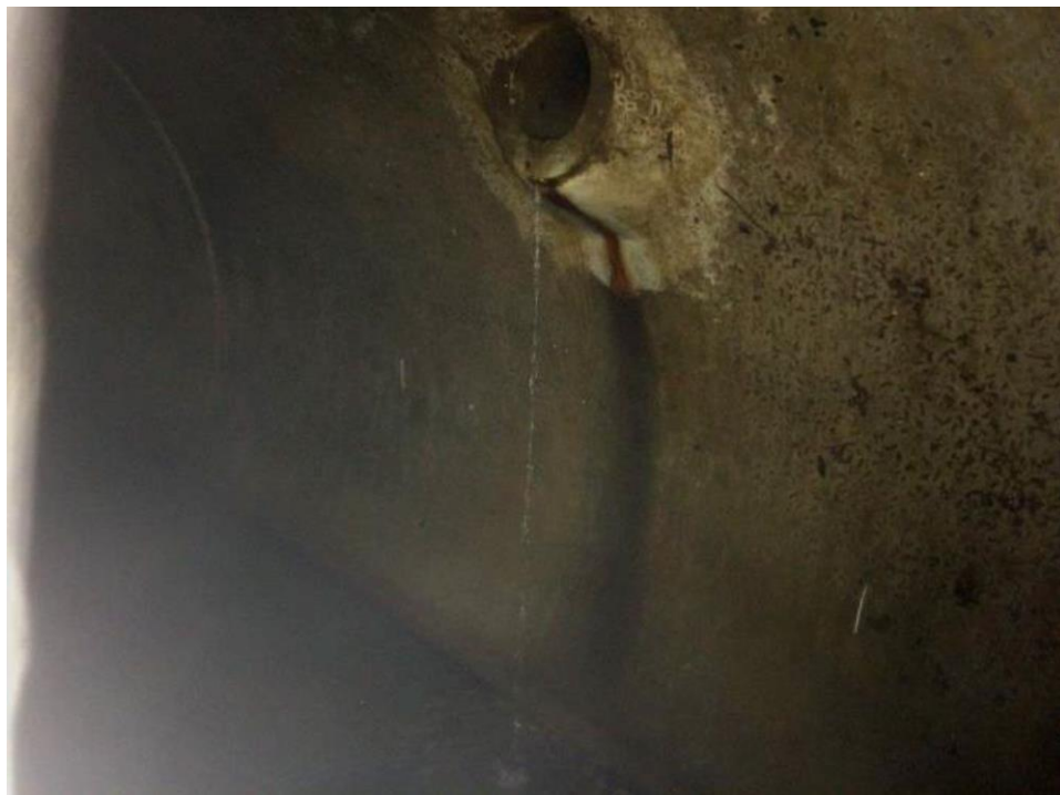
Photo 1: View of a wastewater network overflow pipe into a stormwater pipe that discharges to the CMA (Source: WWL response to further information request email dated 4 May 2018)
