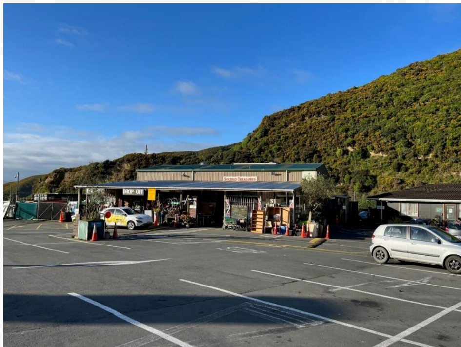
Figure 4 – Tip Shop and staff facilities
