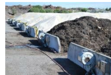
Figure 5-1 Timaru composting facility
