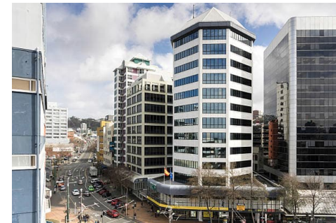
Figure 3-14 Wellington City commercial buildings
