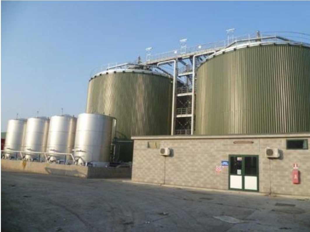
Figure 4 – example of wet anaerobic digestion facility
