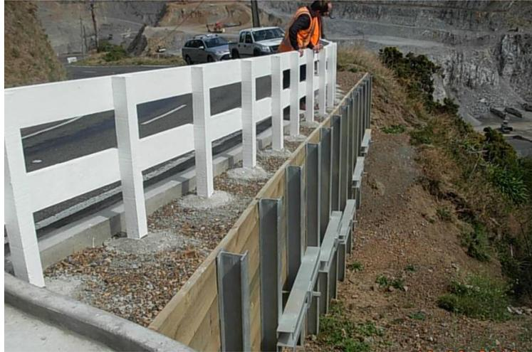
*Figure 11 Horokiwi Rd (anchored steel pole)*
