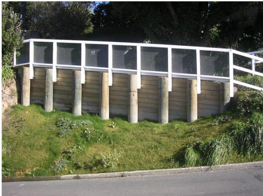
*Figure 19 The Drive (Cantilevered timber pole)*
