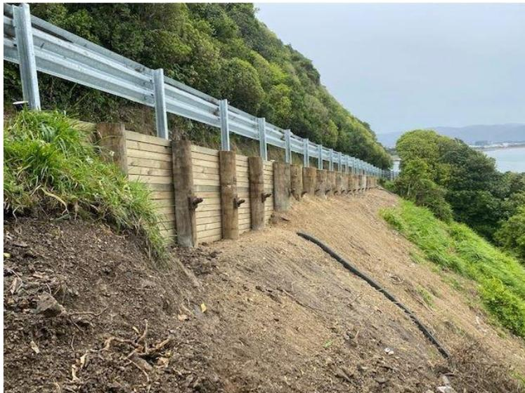
*Figure 12 Horokiwi (anchored timber pole)*
