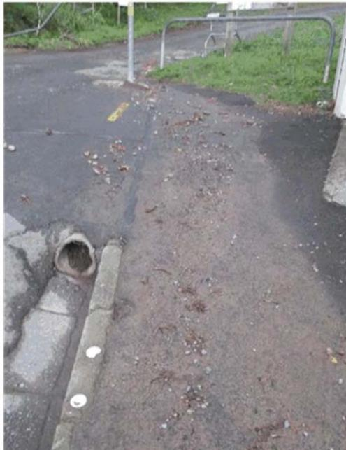
3. Reinstatement of the paved area in the Town Belt between Ellice Street and the old Quarry site. The area was once sealed. It is now covered in large pot holes and strewn with rubble. The rubble gets carried down into the storm water system. Resealing the area will help
