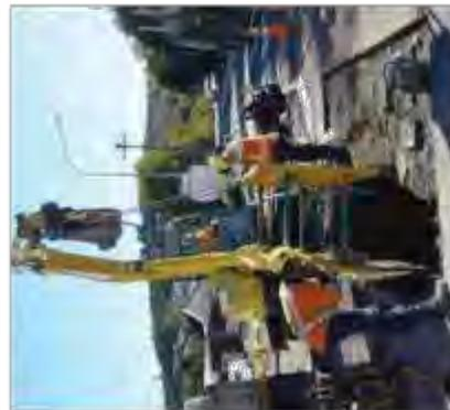
Workers lower shoring components into a trench for a project in Upper Hutt. The trench heights at which shoring must be in place have been reviewed by Wellington Water recently, to ensure workers performing tasks below ground level are safe.
