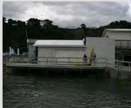
The PD shed and walkway to the beach is constructed (2009)
