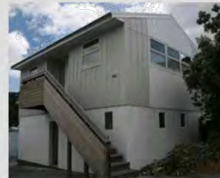
The changing rooms are refurbished after 30 years of hard use (2013)
