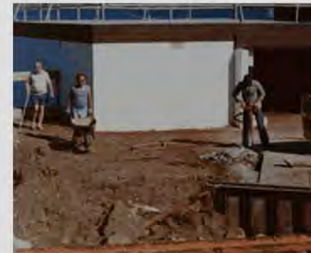
Building changing rooms, rescue boat shed and extra hardstand (1980-1985)
