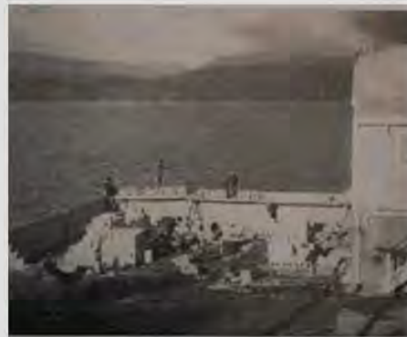
Members putting up the walls of the North shed (1970)
