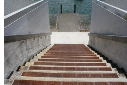
New step caps and handrails
