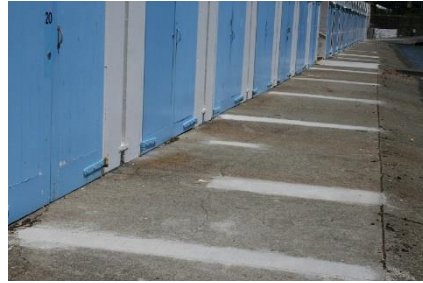
Patching of cracks in concrete
