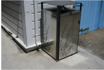
Install of new rubbish bins
