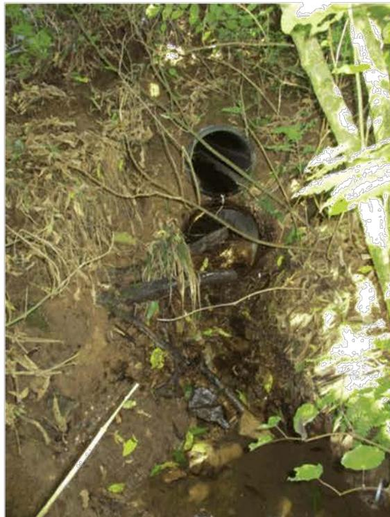
Plate 6: Double culvert under a section of the existing access track. 29 March 2019.
