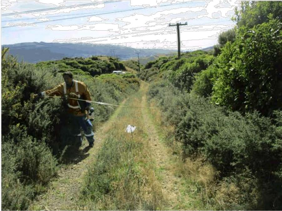
Plate3: Measuring tape showing a four metre width of a section of the access track that would be used to install the 11kV cable underground . 29 March 2019.
