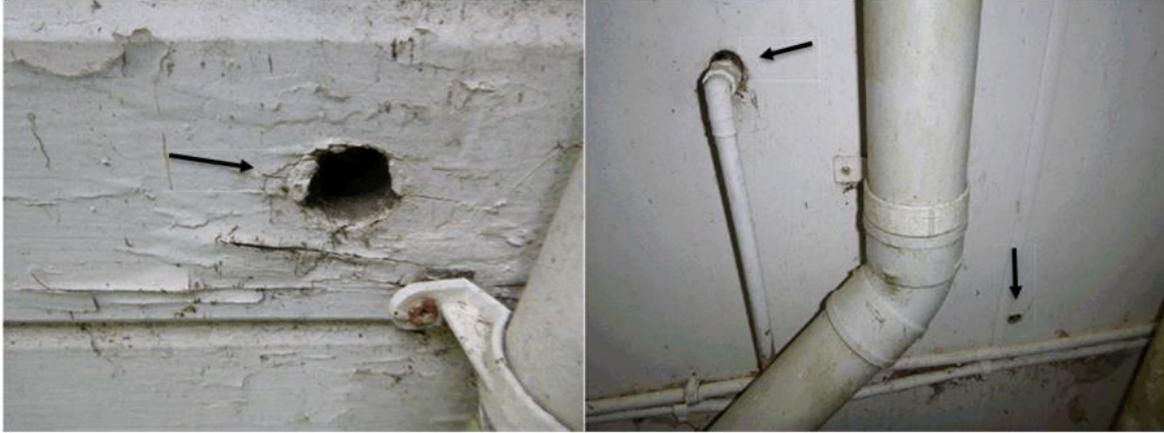
All penetrations should be plugged and sealed to the cladding prior to the next decorating period.
