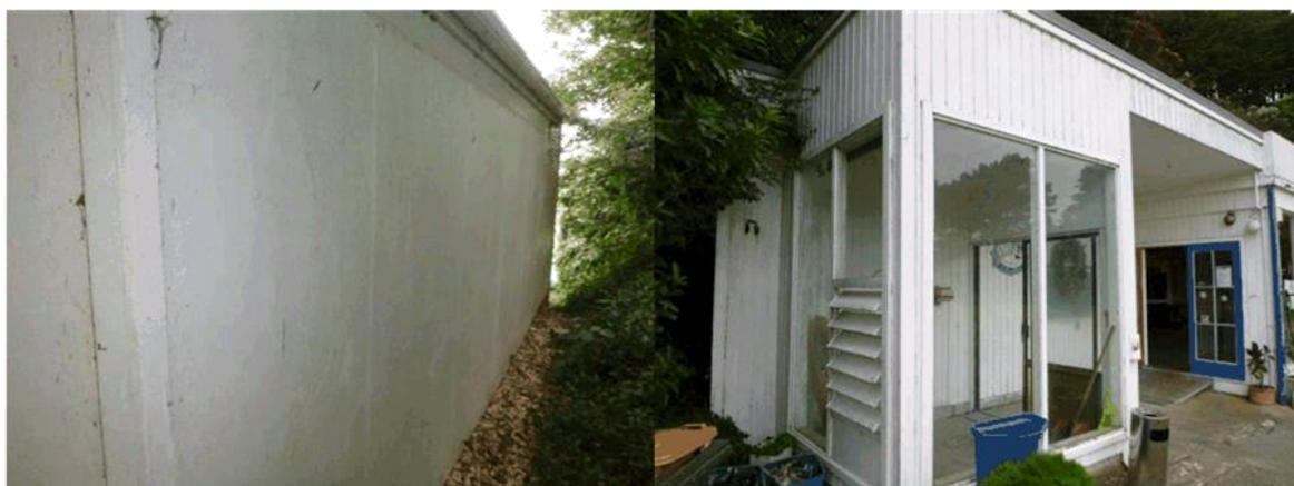
The exterior of the building is multi-clad with the use of timber weatherboards and a profiled fibre cement asbestos sheet.
