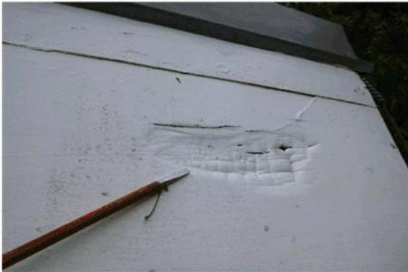
Above is the southern end of the front barge board that shows a small section of decay. This could be removed and replaced with a new section and painted.
