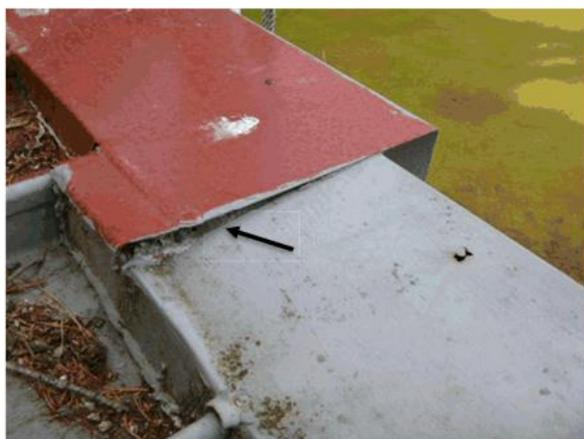
The barge overlap should be a sealed junction.
