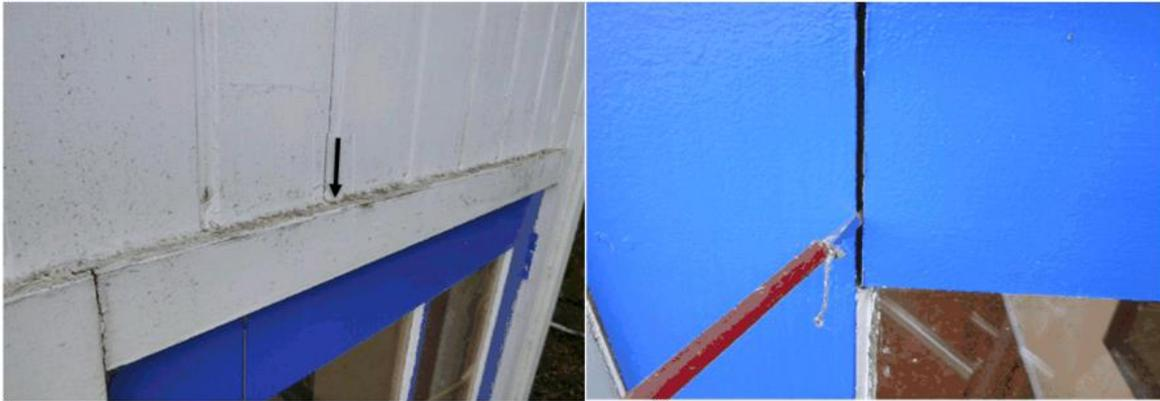
The far-right exit door frame could have a head flashing installed above the joinery opening to add further protection. The door itself through age shows some movement in the rail/style connections which could be glued (using a water proof high strength building adhesive) clamped, and then painted.
