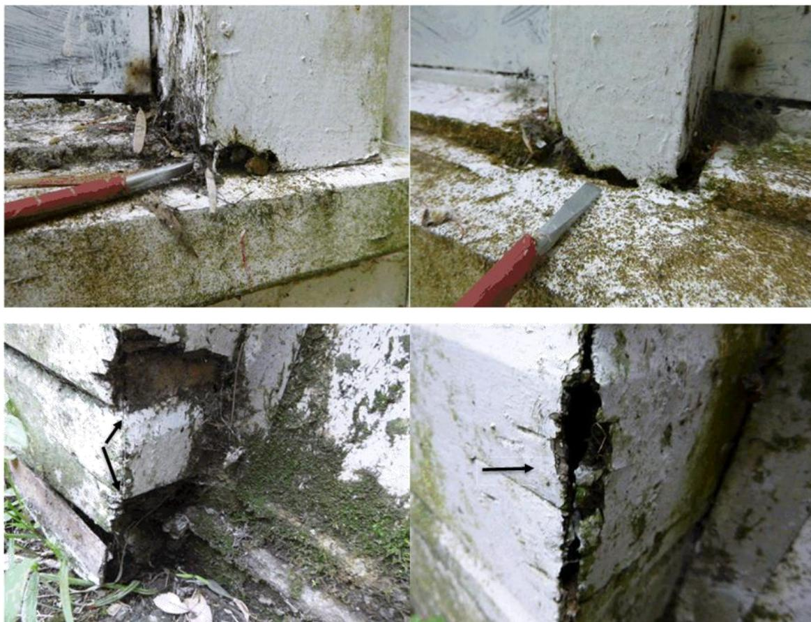
To the rear south eastern side of the building there are a few areas that show general wear and tear on the weatherboard and architrave components that could be tidied up with sections replaced as required and mitred corners could have a corner soaker installed over them to seal and improve the aesthetic appearance.
