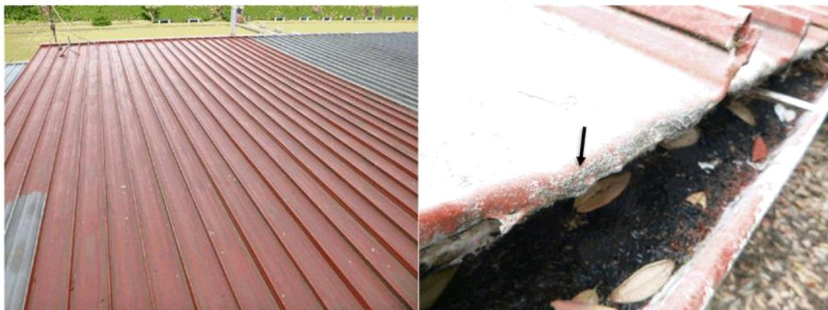
The main roofing is a very flat roof profile with the ends of the trough sections turned down to the gutters.
