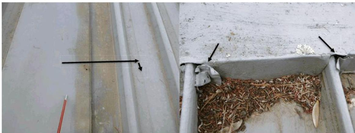
At the northern end where the original main roof meets the next section added, the cover flashing is loose and not properly fixed down to the roof sheets as well as only covering one trough ridge instead of two. It is recommended that this be replaced and to cover two ridges where there is a point to then fix to.
