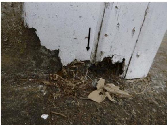
The west facing side of the store room could have head flashings installed over the top of the window and door openings as is customary. Both the architrave trim and boxed corners show decay that could be replaced in part of whole.
