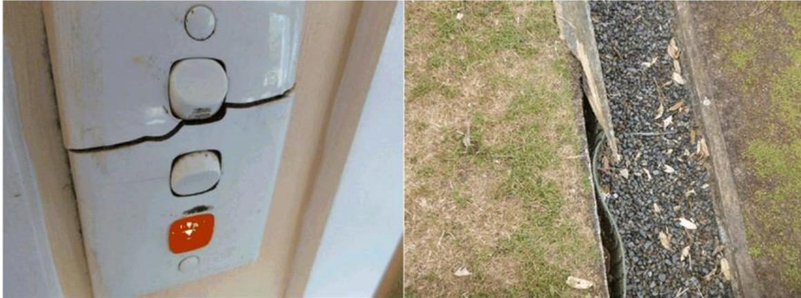
Consideration to replacing light switch face plates is a good idea. On the greens some maintenance to the surrounding edging could be undertaken if not to at first remove any sharp timbers.
