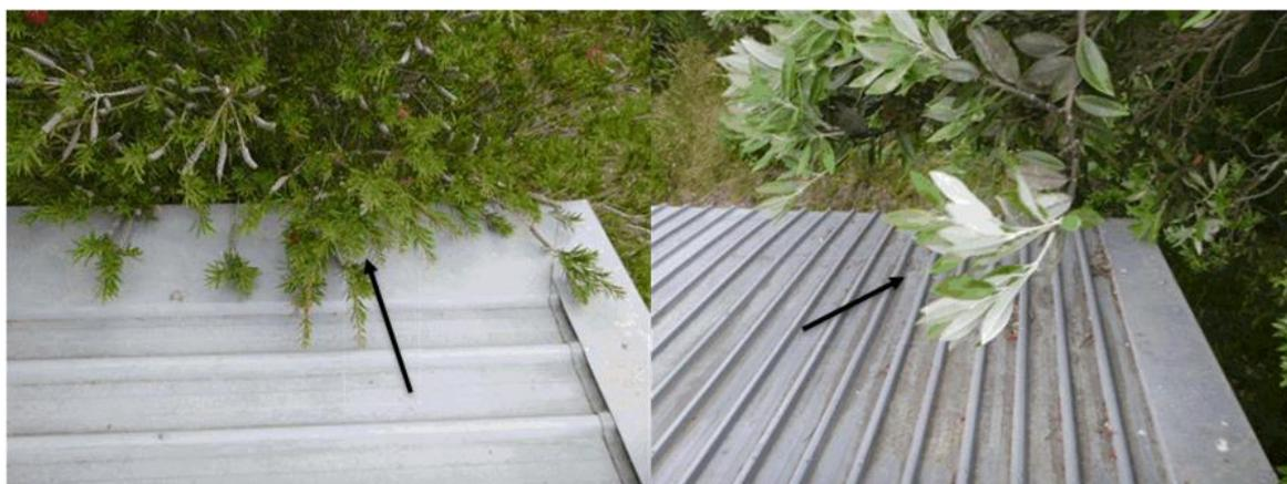
On the southern end extension, the trapezoidal roof profile shows some minor surface corrosion to the ridges and surfaces of one smaller section beneath the tree-line. This should be treated with a rust converter and painted to apply a further protection. The treeline and shrubs need to be trimmed back to prevent premature wear to the roof surfaces.
