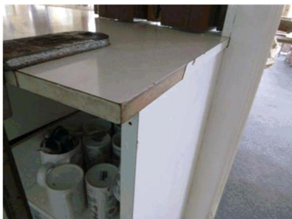
The kitchen could have some further maintenance scheduled to various items. This could include the clashing strips on the bench edges, painting the ceiling and having an electrician place the lighting connection into a junction box.
