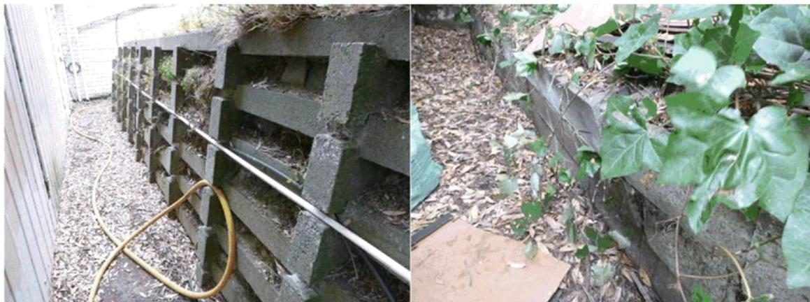
The main crib retaining wall is in good overall condition with no rotation. At the rear, east side of the building the low concrete block retainer has slipped forward over time. This could be removed, the bank cleaned up and the same wall reinstated .
