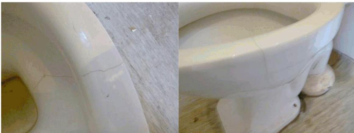
The toilet pan is cracked and it is recommended that it be replaced.
