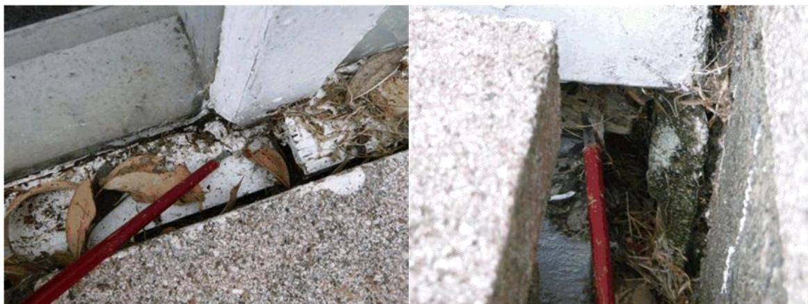
The front timber joinery areas show some deterioration around/on the glazing beads and architraves in each window section. The worst affected ones could be the starting point, being removed, seal rebates and reapply new architraves and beads. During the process it may also be a consideration to apply, prior to reinstating new beads and architraves, Metalex, Concentrated Timber Preservative.
