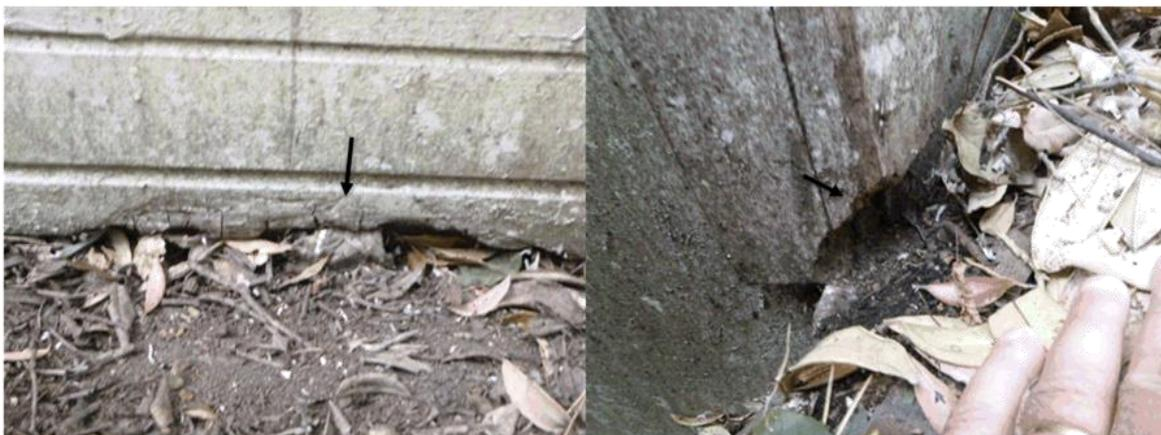
To the rear walls, the weatherboards show some decay to the underside of the lowest board where it is in close proximity to the ground surfaces. Such boards could be replaced either in part or whole. The northeaster corner shows some decay to the base of the boxed corner that could also be replaced. The leaves and residual soil off the bank needs to be cleared away from the cladding surfaces and components to stop the transfer of moisture over prolonged periods.
