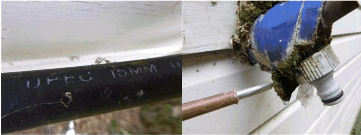
The water pipe to the building is a combination of copper, grey Buteline Polybutene and black Buteline Polybutene. There was no sign of the black Dux Qest labels and the pipe installed here is considered suited for purpose. There is a leak to the tap at the rear southern wall that could be repaired.
