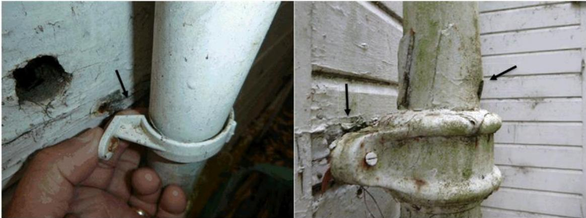
Loose and missing pipe brackets need to be installed and secured. I note the terminal vent pipe needs to have a sleeve installed and a breather cap at the top of the pipe.
