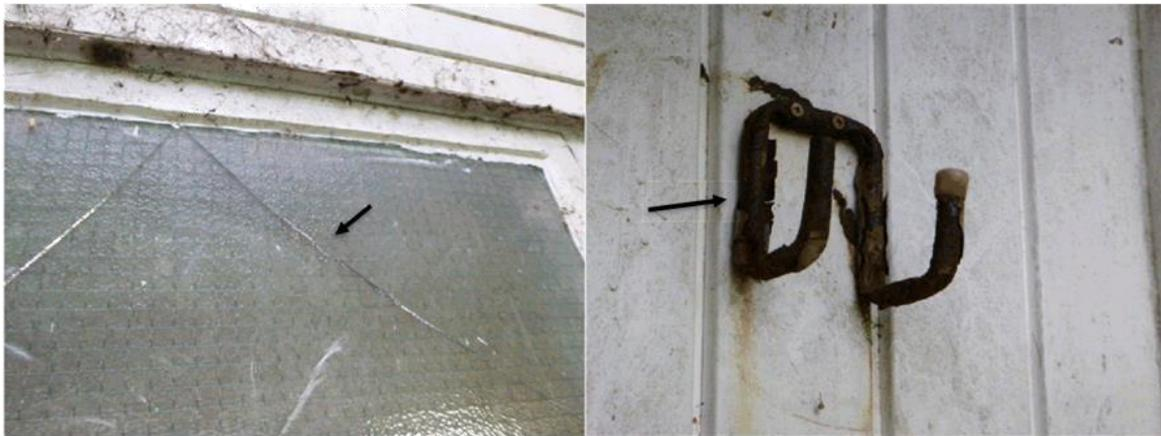
Any pane of cracked glazing could be replaced. Rusting fitting could be removed and replaced as may be desired.
