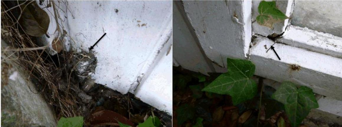
Northern side of the store room shows some decay at the base of the weatherboards that are close to the retained area as well as to the adjacent window sill and trim on the left corner.
