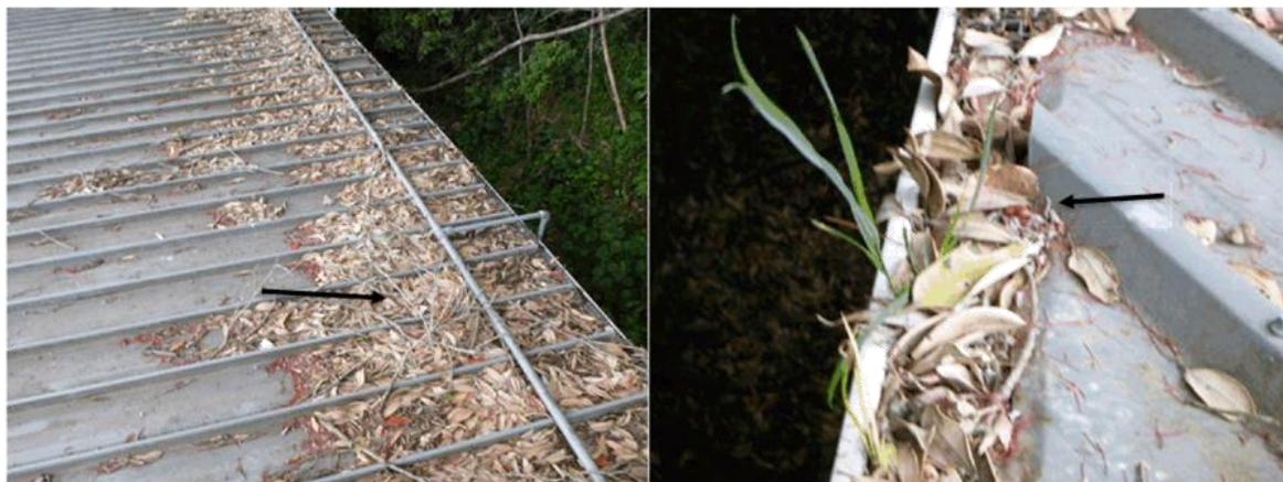
The roof and gutter systems need to be cleared of obstructions and plant life in order to appropriately function.
