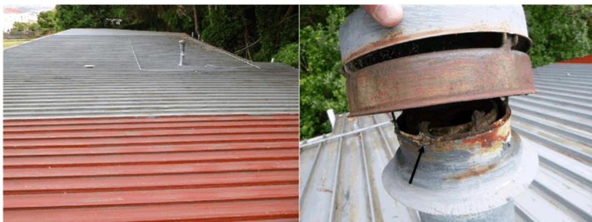
The roof could be re-painted to add a further film of protection at some stage. The cowl to the flue shows corroded bracket stays and is loose, which could be replaced.
