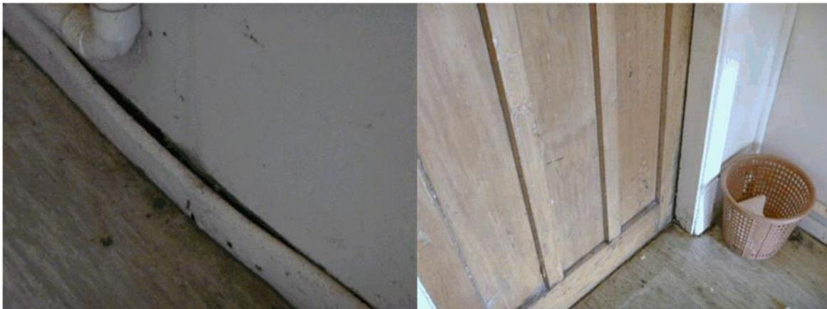
Skirting boards can be tacked or glued back to the wall linings. The rear door is binding a little and could be eased.
