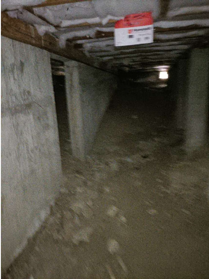
Typical interior concrete foundation wall
