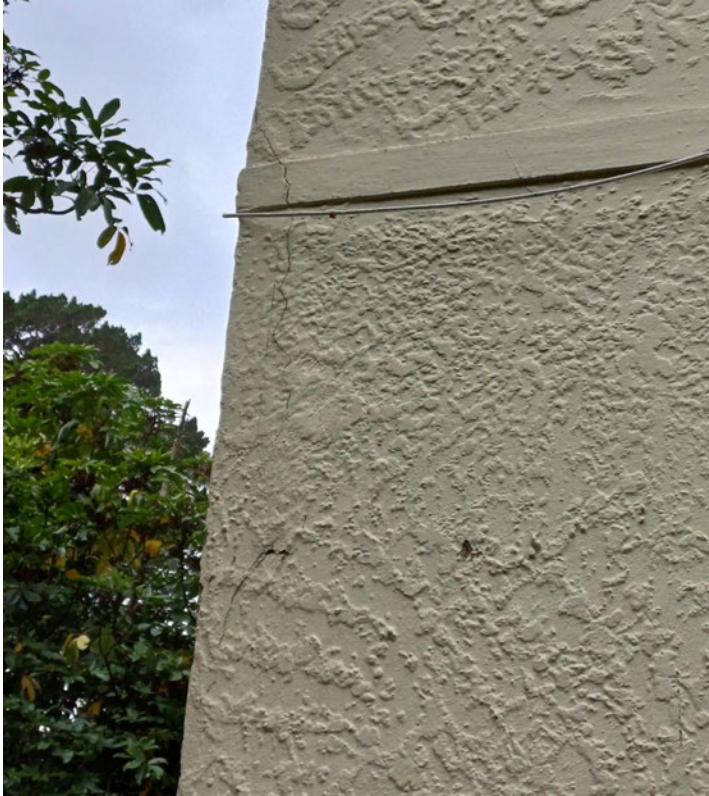
Cracking at Glenmore/Driveway Corner (Grid F/5 intersection)
