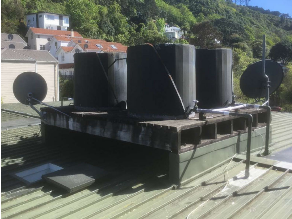
Figure 13: Roof tank support structure
