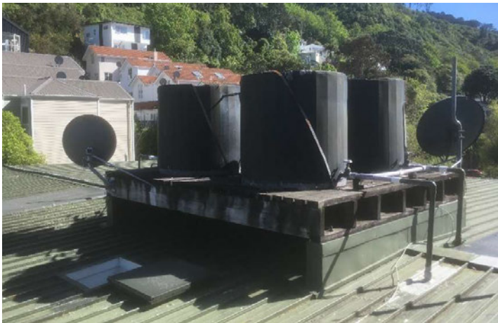
The tanks at roof level are supported on a timber platform with no apparent seismic system.
