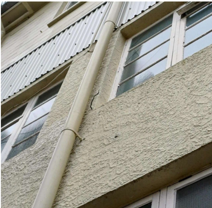
Cracking on Grid 1 pier.
