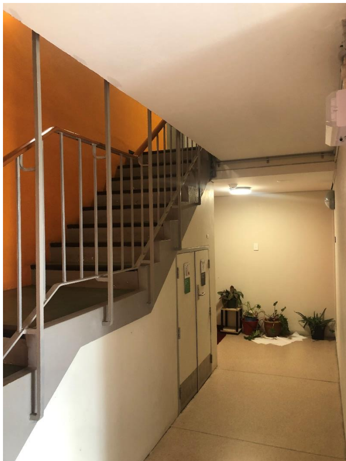
Photograph 2: Internal concrete stair
