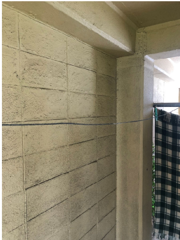
Photograph 2: Blockwork infill wall
