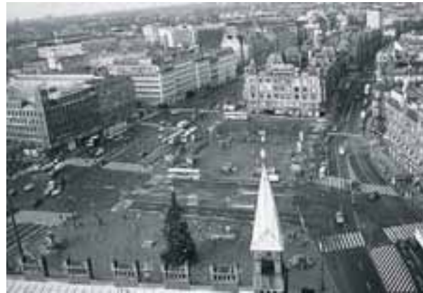
Above: The Town Hall Square in 1995 before renovation when traffic divided the square in two separate parts. The Town Hall Square was renovated when Copenhagen was the European Cultural Capital in 1996.
