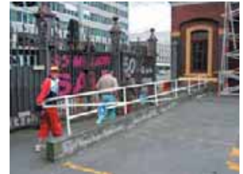
Some entrance points suffer from poor quality and lack of attention to detail.
