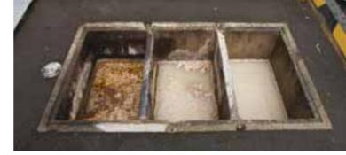
Passive grease traps cool down waste water so fats and oils float to the top.
