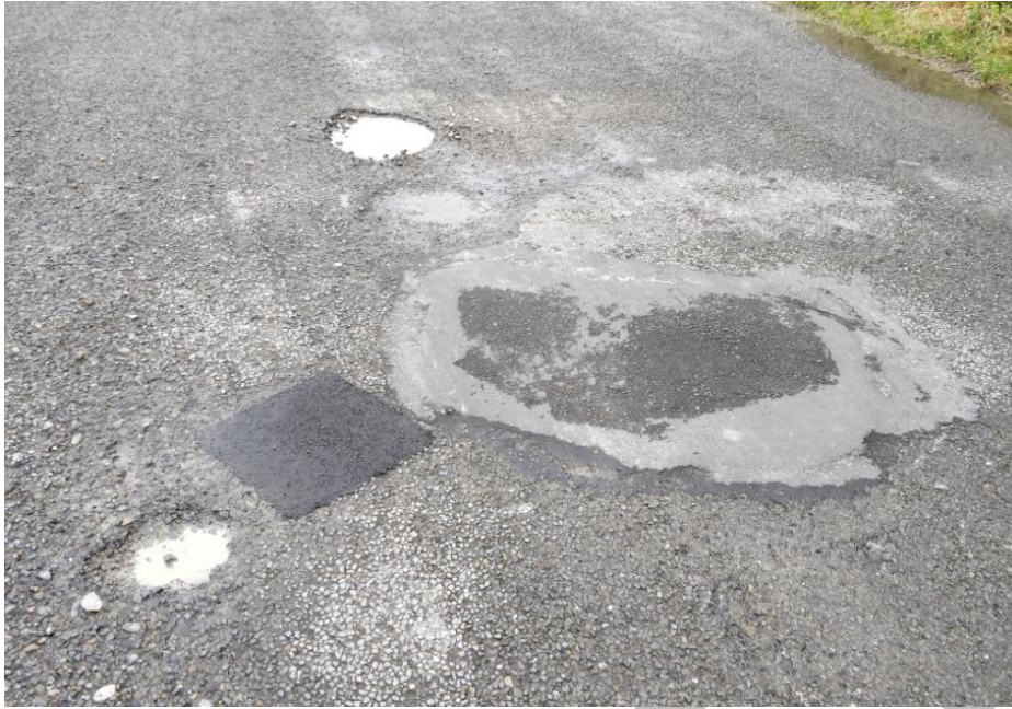
Figure 4-3: Typical example of potholing in Section B
