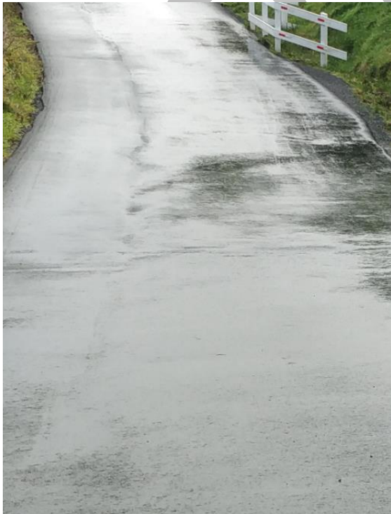
Figure 4-4: Recent AC pavement repair on Section B (Near wind turbine)
