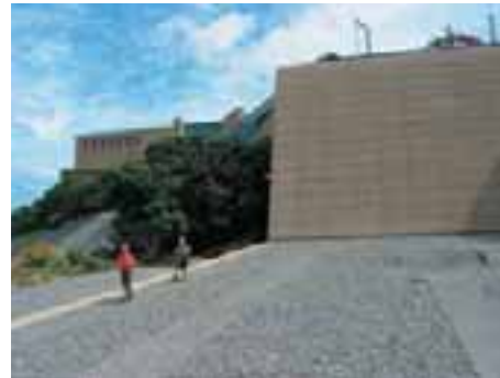
Te Papa's exterior is defensive and takes little advantage of a prime location adjacent to the water's edge.
