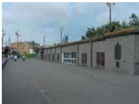
Most facades along the waterfront are closed and uninteresting.
