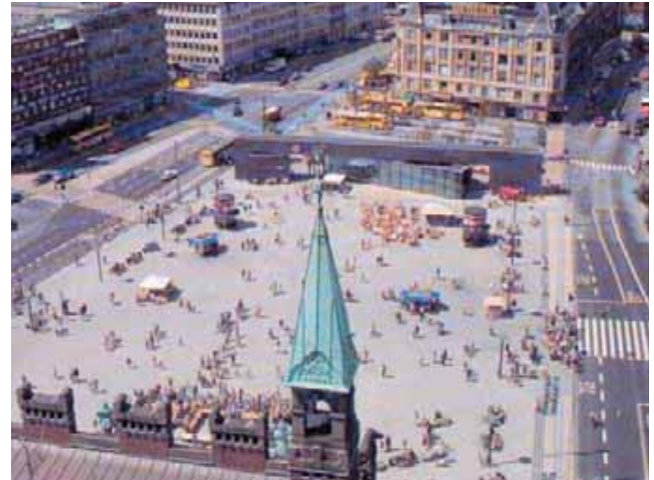
Renovation turned the Town Hall Square into a large unified bowl-shaped space defined by a pavillion building in dark glass.
