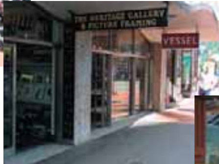
B Pleasant Relatively small units (10-14 units per 100 m) Some diversity of functions Only a few closed or passive units Some relief in the facades Relatively good detailing
