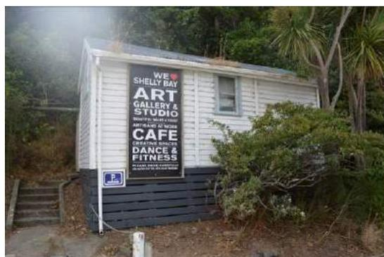
**Fig. 65** View of the outbuilding looking towards the south elevation. Note the concrete steps which provide access up to the main entrance and rusticated weatherboards on this elevation.
