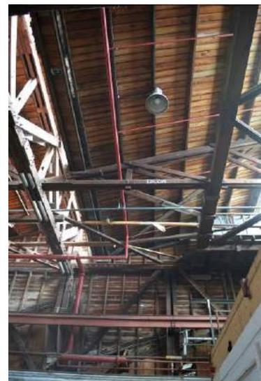
**Fig. 86** View of the timber roof structure. Note the wide span ladder trusses, heavy gauge structural timbers, exposed purlins and sarking.
