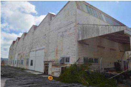
**Fig. 77** View of the west gable, high stud portion of Shed 8. Note this elevation directly addresses, and links to, the wharf structure.
