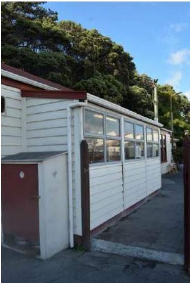
**Fig. 95** View of the non-original lean-to structure constructed on the against the veranda on the north-western elevation. This forms additional kitchen facilities.
