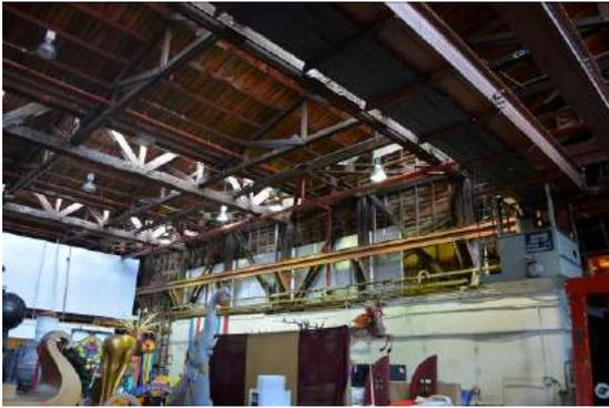
**Fig. 87** View looking west across the high stud double storey section of the building. Note the timber roof structure with wide span ladder trusses, heavy gauge structural timbers, exposed purlins and sarking.
