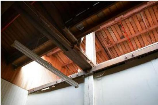
**Fig. 82** Looking above internal non-structural partitioning to view the timber roof structure.
