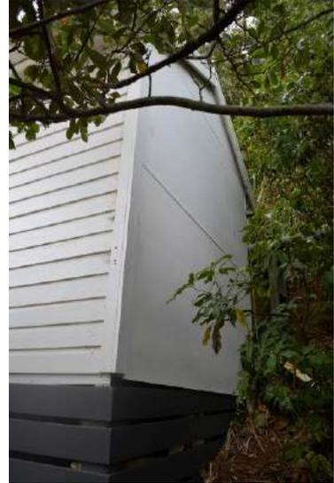
**Fig. 68** View of the east gable. Note the flat sheet material used for the cladding.
