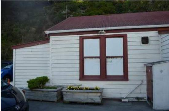
**Fig. 93** View of the pair of double-hung sliding-sash windows (boarded up) in the north end of the principal elevation.
