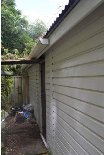
**Fig. 67** View of the main entrance door in the north elevation. Note the rusticated weatherboard on this elevation.
