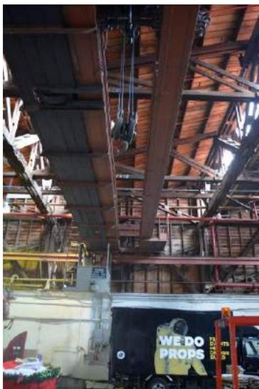
**Fig. 85** Interior view looking east across the high stud double storey section of the building. Note the gantry crane remains in-situ.
