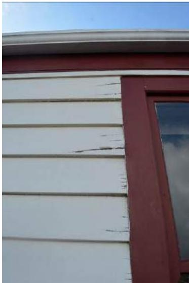
**Fig. 99** Evidence of decaying weatherboards.
