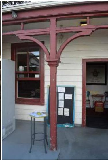
**Fig. 97** Note original braced posts and timber fretwork.
