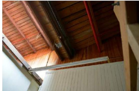
**Fig. 83** Looking above internal non-structural partitioning to view the timber roof structure.
