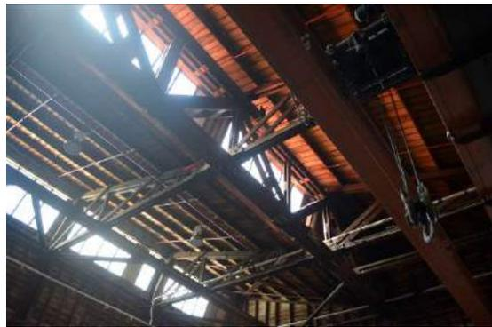
**Fig. 90** Looking back towards the south aspect. Note the glazed portions of the saw-tooth roof profile.
