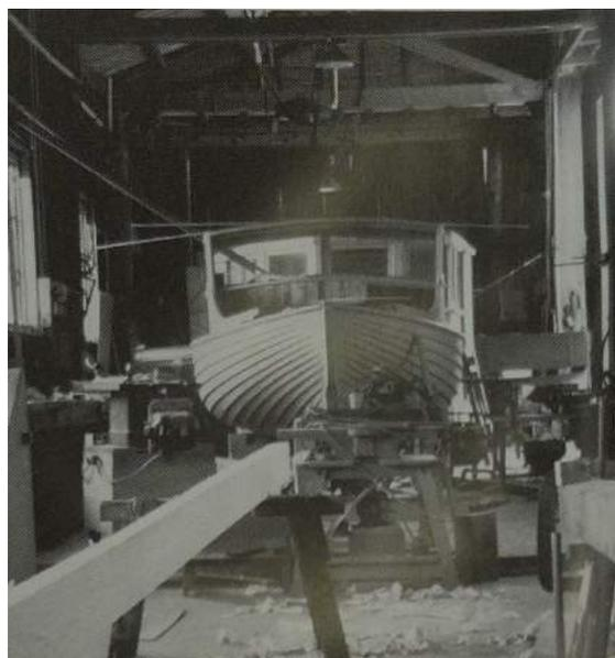
**Fig. 19** Two views looking north within the Shipwright's Building in the 1950s, showing boats under construction and repair. Note the monopitched roof, with half-truss roof structure. (Berthold, "B.T. Daniel Ltd., Shipwrights, Boatbuilders & Marine Engineers, Shelly Bay, Wellington," *New Zealand Marine News* v.58, no.1, p20)
