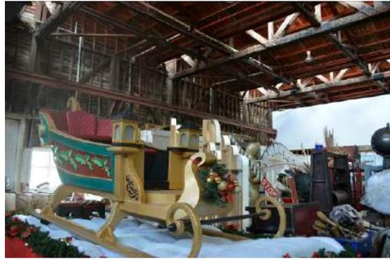
**Fig. 88** View looking towards the west elevation, across the high stud double storey section of the building. Note the timber roof structure with wide span ladder trusses, heavy gauge structural timbers, exposed purlins and sarking.
