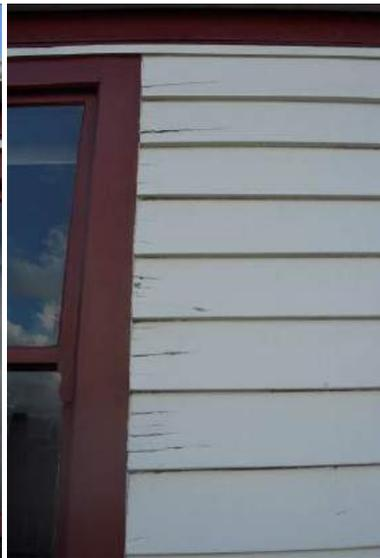
**Fig. 100** Evidence of decaying weatherboards.
