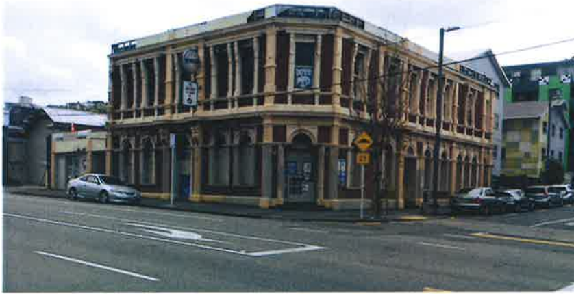
Photo 1: former Tramway Hotel, 114 Adelaide Road, Mt Cook
