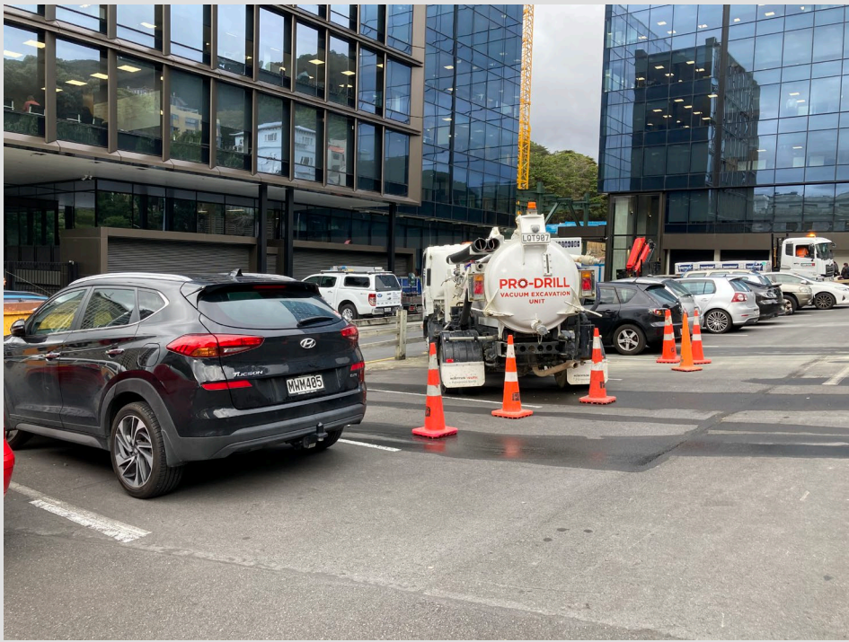
Figure 3 Site – Facing South-West
