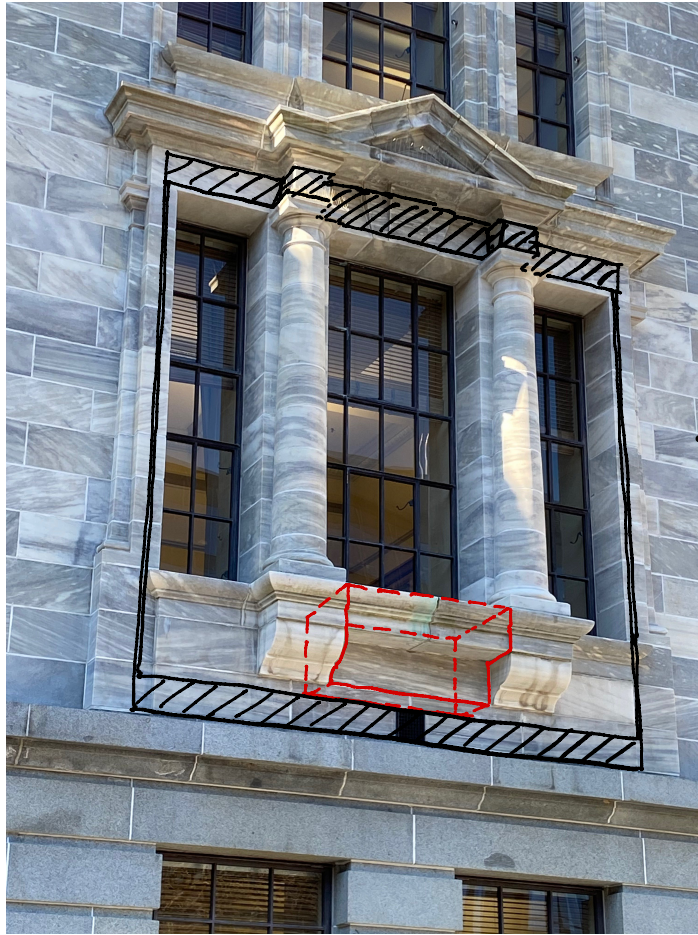
Figure 11. Showing the 3-part window where the link bridge will enter. The red line indicates where the stone is proposed to be cut away. The black line shows approximately where the bridge link will make contact with the facade.
