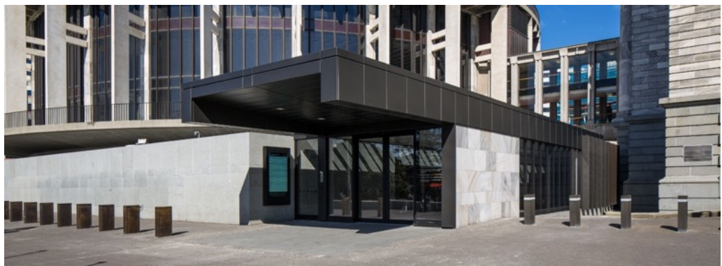
Figure 14. Photo of front entrance showing composition of a metal cladding with a lighter coloured base
