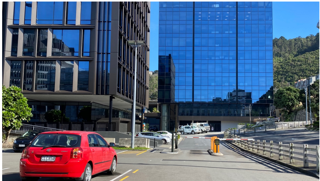
Figure 13. Photograph showing the ground floor of the BSB and CFT at Ballantrae Place
