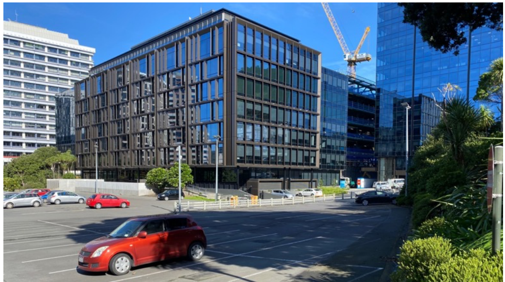
Figure 7. Looking across the western carpark to the Bowen State Building with the Charles Fergusson Tower on the right.
