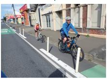
Flexi-bollards, either individually bolted to the road surface or set into a ground separator which is then bolted to the surface.
