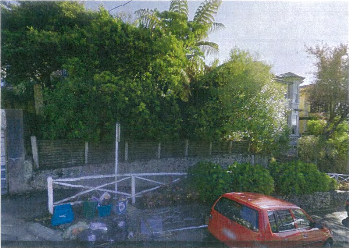
View of 12 Essex Street from Essex Street
