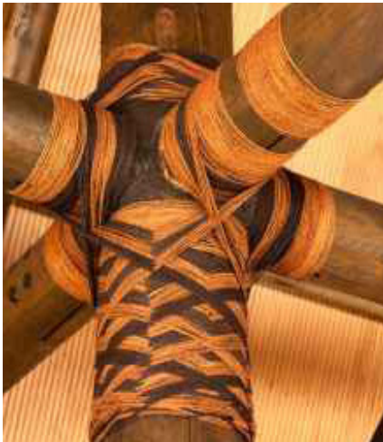
1.6- Structural connection joint that expresses a new ‘lashing’
