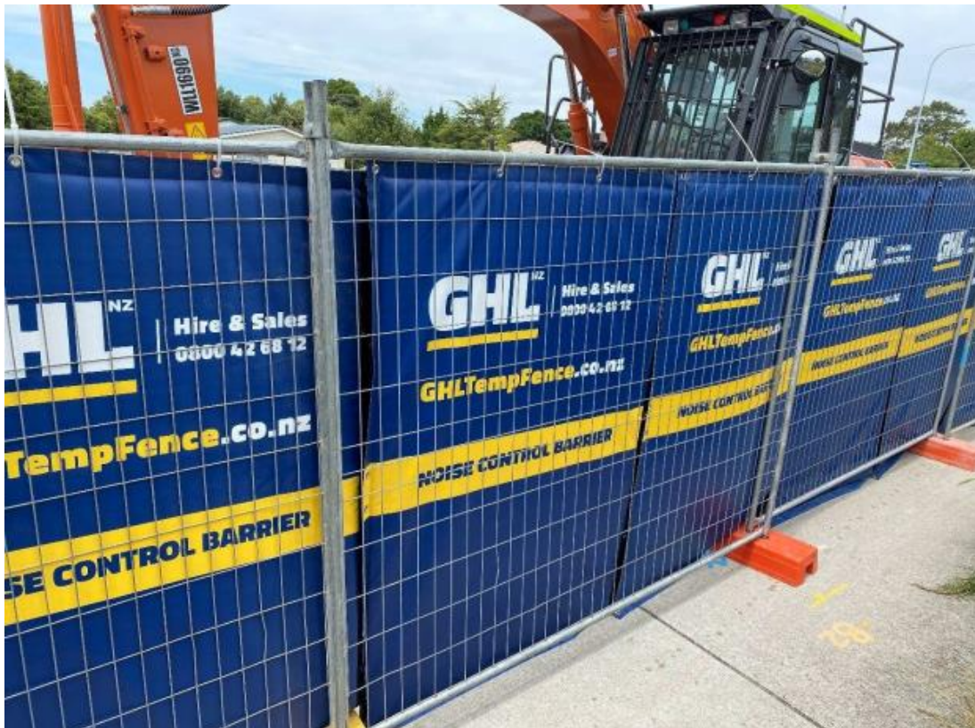
Figure 7 Example of Localised Acoustic Screening (minimum 2.0m high)
