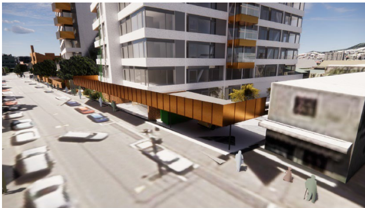
FIGURE 2 1.5M UPSTAND ON THE CANOPY AROUND THE SOUTHERN BUILDING (FROM DECEMBER 2021 ATHFIELD ARCHITECTS ILLUSTRATION IN WIND – CANOPY DETAILS.PDF)
