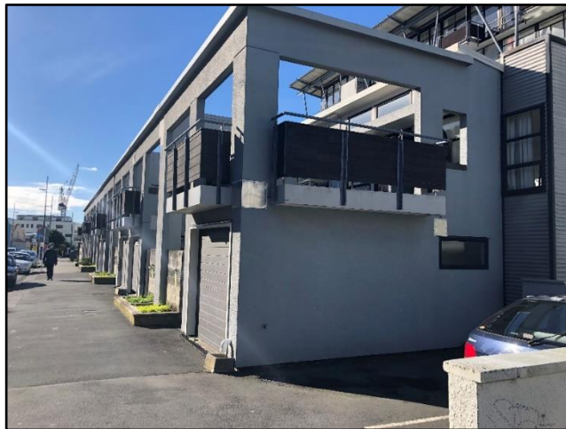
Figure 3: Taken looking north along part of the Tasman Street frontage of 23 Tasman St
