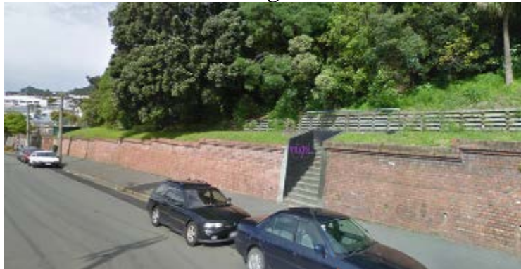
Tasman Street retaining wall – centre
