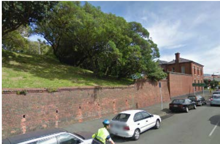
Tasman Street retaining wall – northern end.
