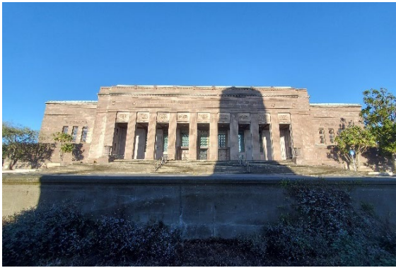
Fig. 23 Looking south from the Carillon and National War Memorial towards the former Dominion Museum.
