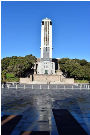
Fig. 20 Looking south across the National War Memorial Park directly along the formal designed north-south axis towards the National War Memorial and Carillon tower.
