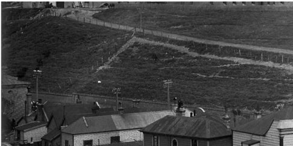
Detail of the retaining wall – note the horse paddocks behind the wall. The wall appears to serve partly as a stock-fence and partly as a retaining wall.
