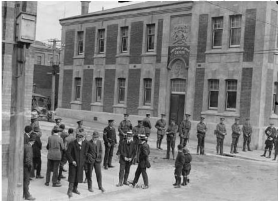
At Buckle Street, Wellington, during the 1913 waterfront strike. Smith, Sydney Charles, 1888-1972: Photographs of New Zealand. Ref: 1/2-048786-G. Alexander Turnbull Library, Wellington, New Zealand.
