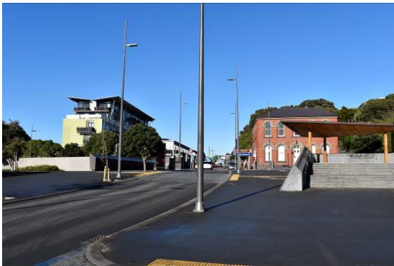
Fig. 10 Looking south along Tory Street towards the intersection of Tory, Buckle, and Tasman Streets, with the subject site (left) and former Mount Cook Police Station (right).
