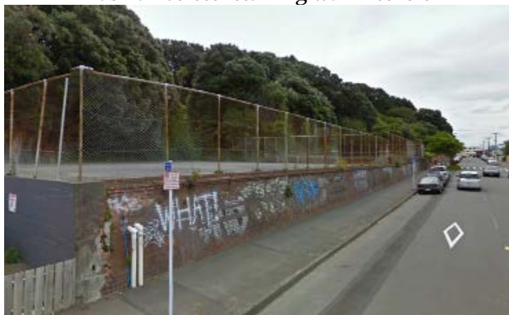
Tasman Street retaining wall – southern end All images: Googlemaps (2009)
