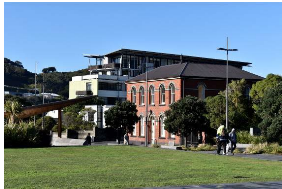
Fig. 11 Looking southeast from the National War Memorial Park towards the former Mount Cook Police Station and the subject site behind.
