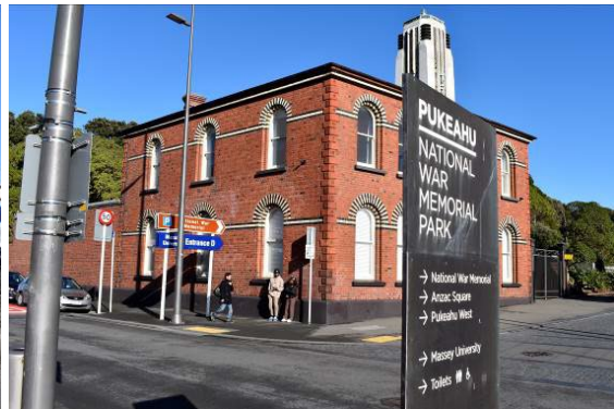
Fig. 13 Looking southwest across the intersection of Tasman and Buckle Streets towards the former Mount Cook Police Station, with the top of the Carillon tower visible above.
