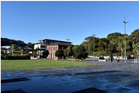
Fig. 25 Looking southeast towards the southeastern corner of the National War Memorial Park bookended by the former Mount Cook Police Station building, with the subject site beyond.
