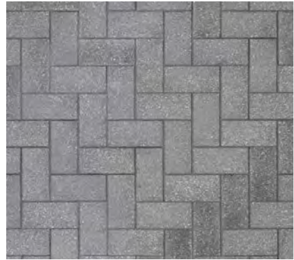
STONE UNIT PAVING
