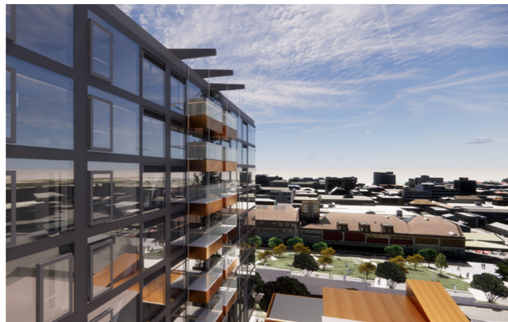
Fig 36. Northern Apartments crystalline facade
