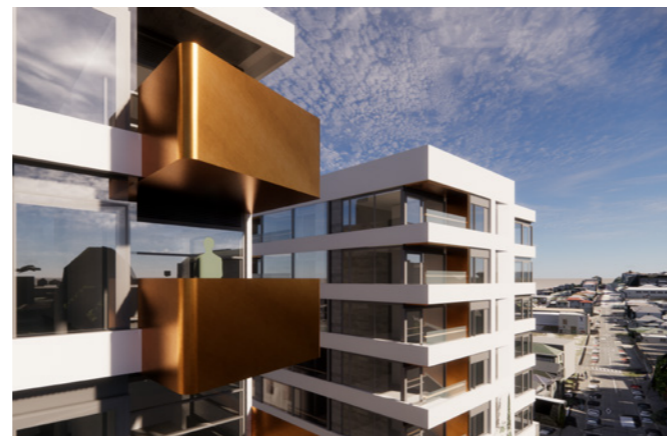
Fig 70. Aerial view of Northern Apartments shaped deck timber soffits
