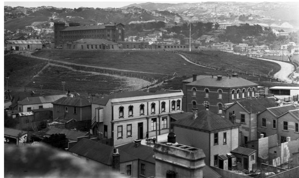
Fig 20. Alexandra Barracks from St Patrick's College Tower (Photograph, 1910, Wellington, by Sydney Charles Smith. Alexander Turnbull Library (1/1-020192-G))
