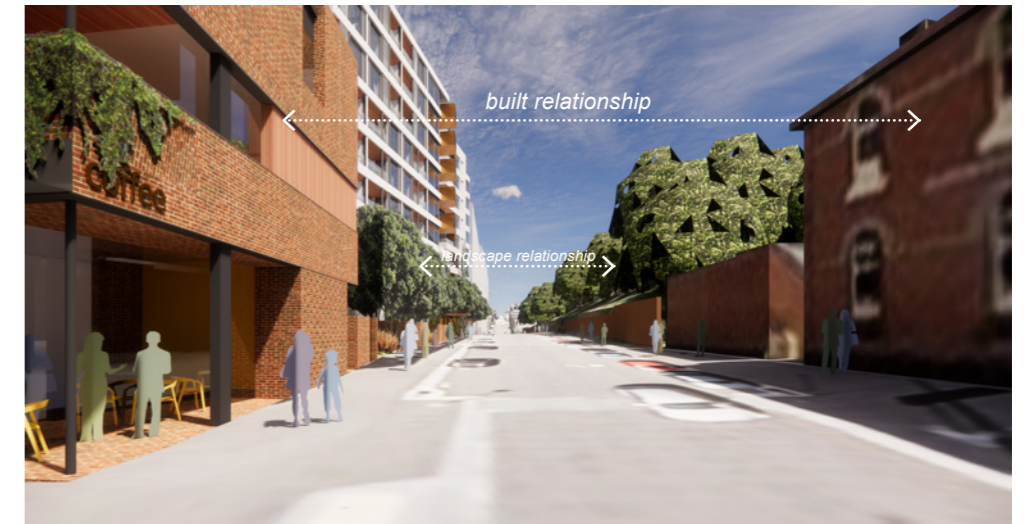
Fig 55. View 04: Looking south down Tasman St from Corner of Tory St and Buckle St
