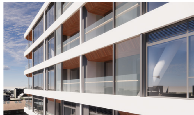
Fig 69. Aerial view of Northern Apartments shaped deck timber soffits
