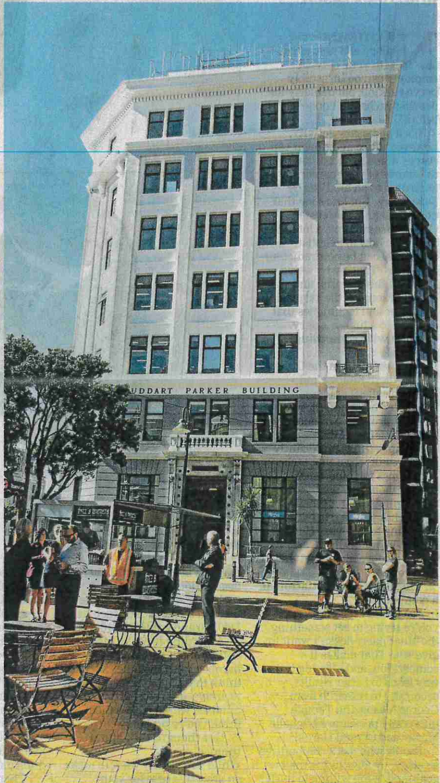
Retro fit: The Huddart Parker building in Post Office Square where almost $9 million has been spent on a major refit and strengthening project.
