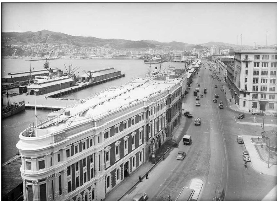
Fig 7: Looking south west over Custom Quay, Wellington. 1/2-042013-G between 1938-9. The Harbour Board buildings are on the left. The Huddart Parker building is on the right.
