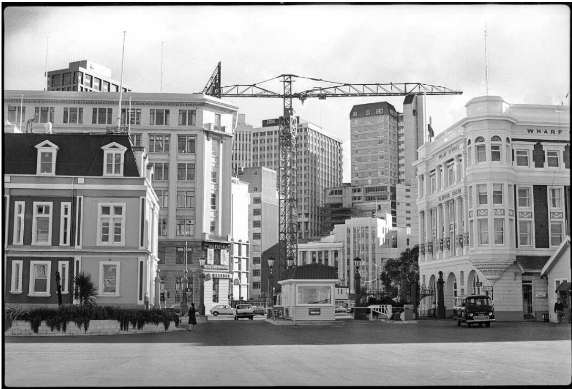
Fig 8 Wellington City from Queens Wharf, 16 July 1977. EP/1977/127/29-F
