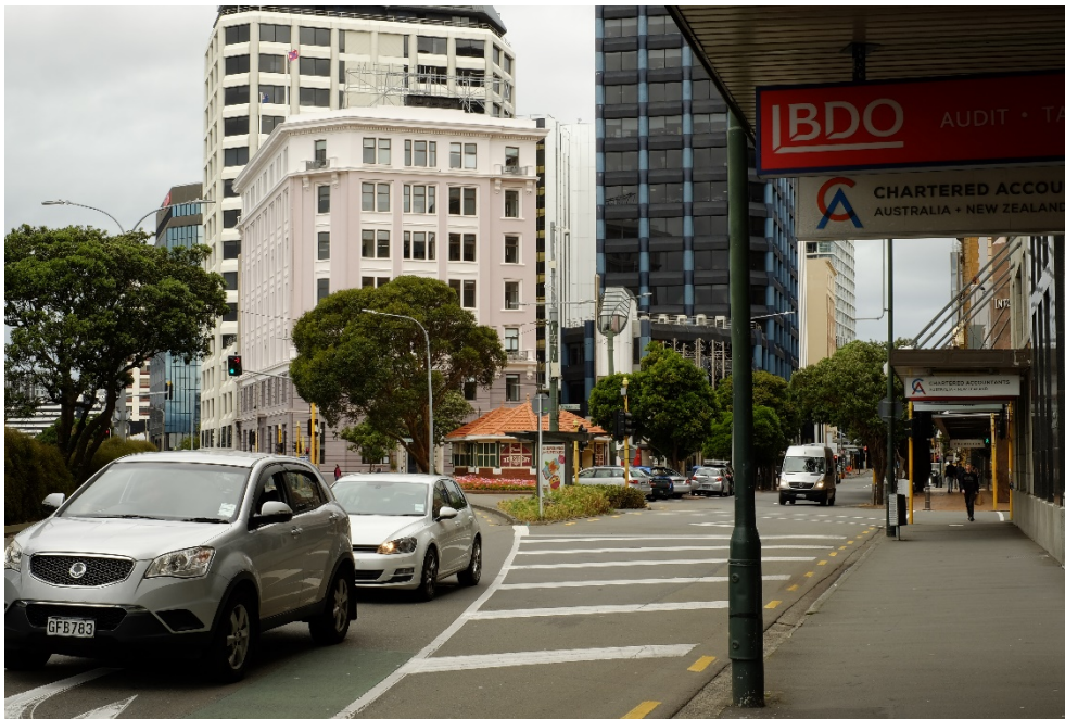
Figure 1: View of the building from the north (from west side of Customhouse Quay)
