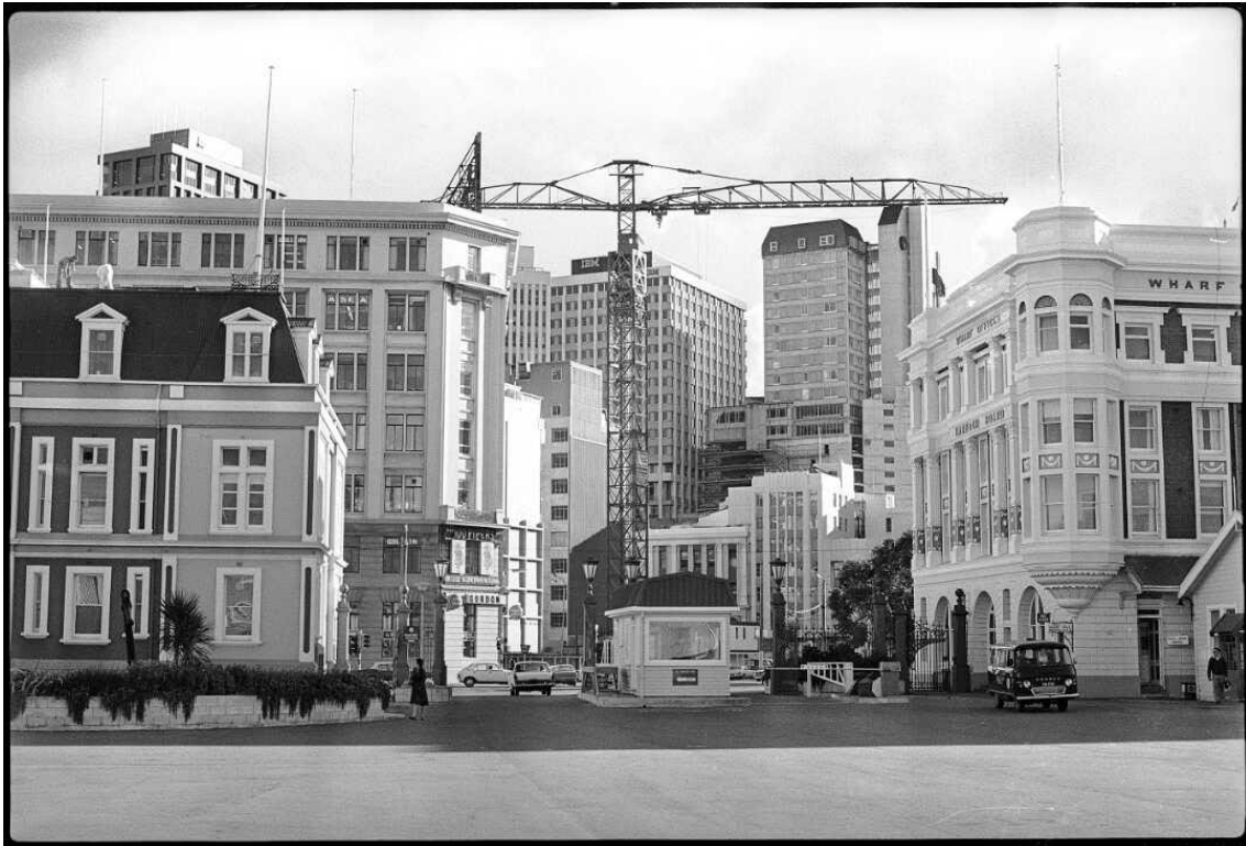
Fig 8 Wellington City from Queens Wharf, 16 July 1977. EP/1977/127/29-F
