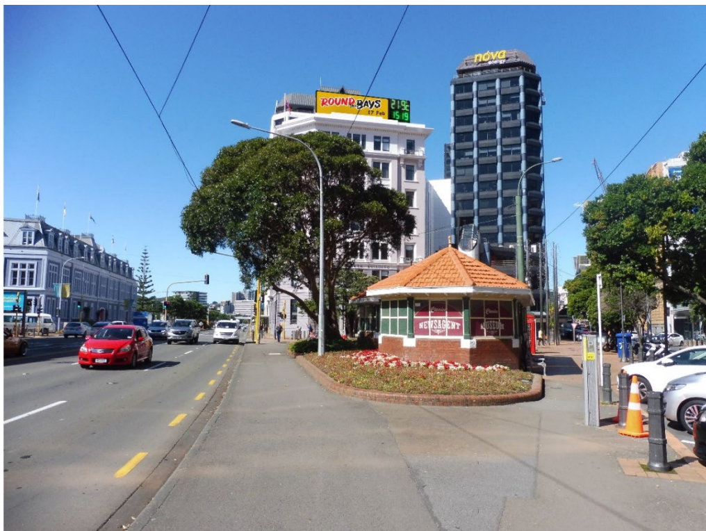
fig. 1 Post Office Square and immediate surrounds (including the Huddart Parker Building) with illustrative' photo montage.
