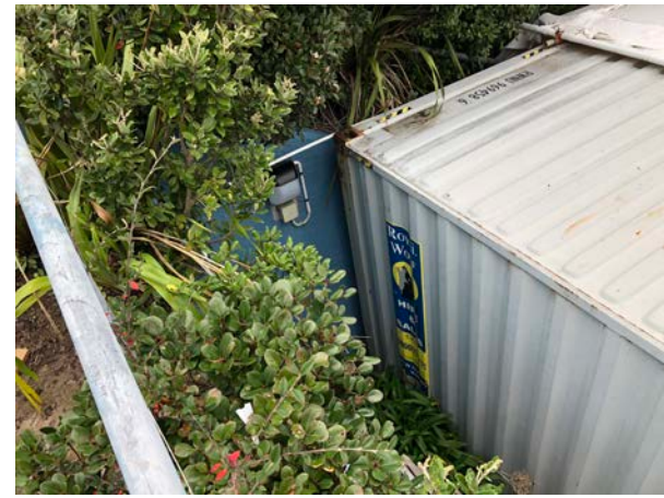
Photograph 6: Retaining Wall and Temporary Storage Containers Along Eastern Boundary.
