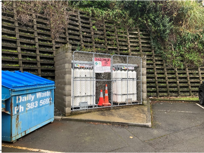
Photograph 1: Oxygenate Tanks Located on Northwestern Corner of Property.
