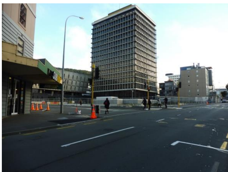
PHOTO 2: vacant site with the 15-storey Freyberg Building to the rear
