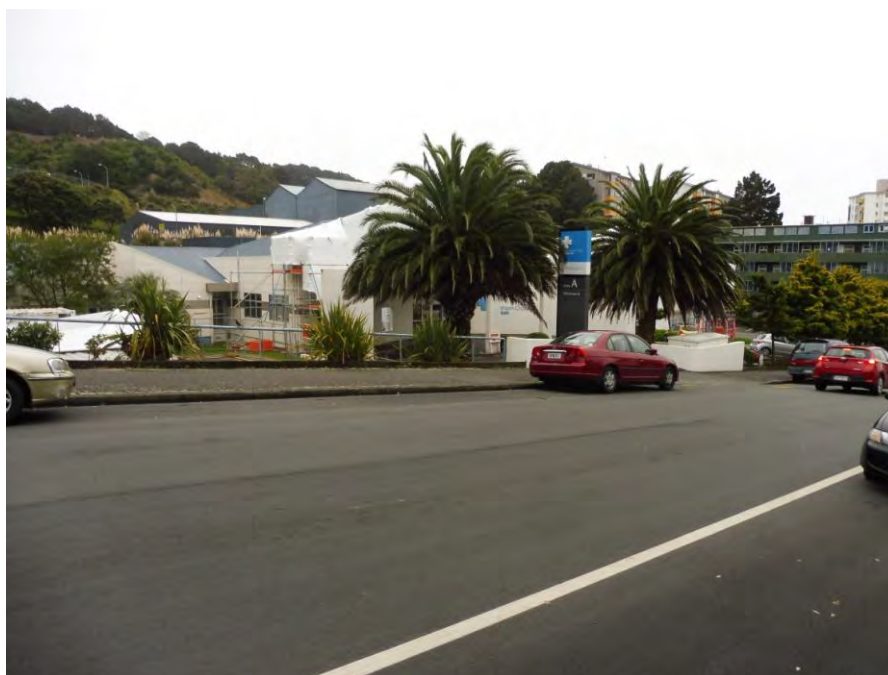
PHOTO 1: Southern Cross Hospital - 90-114 Hanson Street, Newtown
