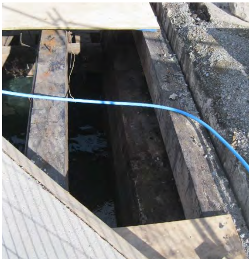
Figure 22: 1901 seawall Concrete edge of seawall visible beneath timber to right O'Keefe
