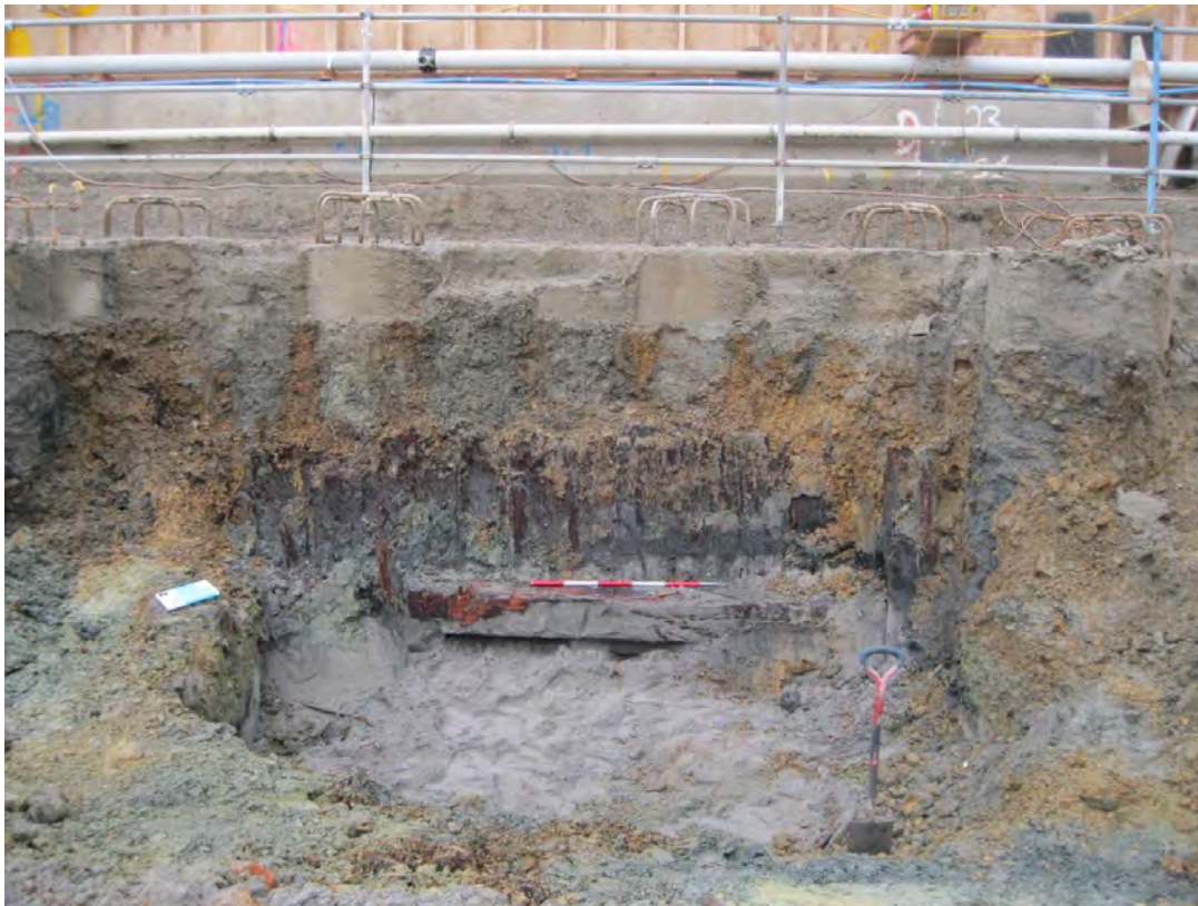
Figure 19: Detail of exposed seawall, bearer, beams and piles visible O'Keeffe
