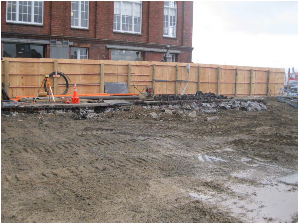
Figure 14: Location of exposed cobbles; north site boundary and Shed 21 in background
