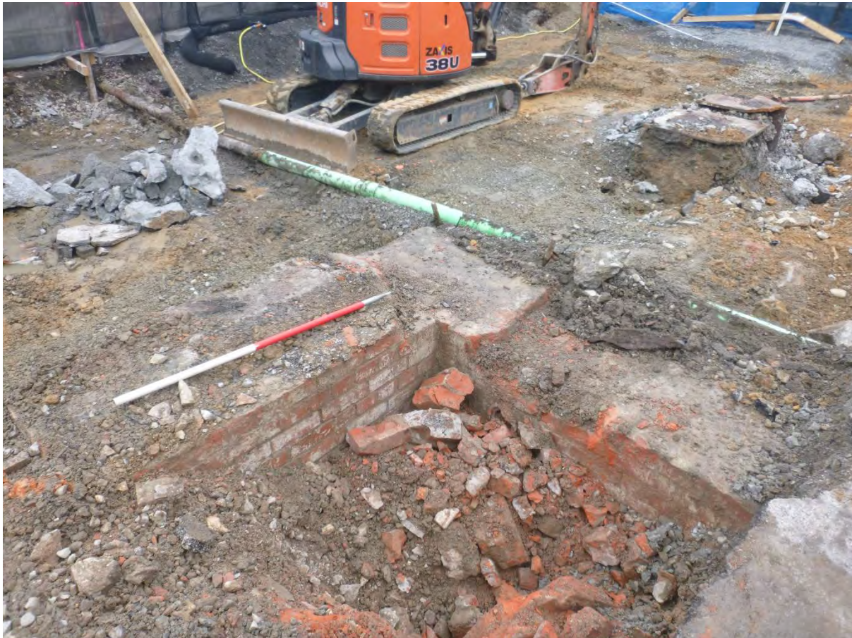
Figure 23: Customhouse foundations O'Keefe
